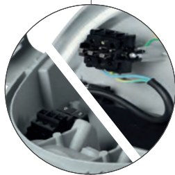
Cut off terminal
